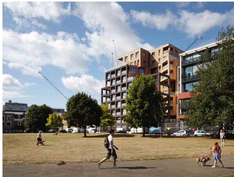
Figura 1. Jack Hobhouse. Fonte: https://www.archdaily.com.br/784367/the-cube-hawkins-brown/
