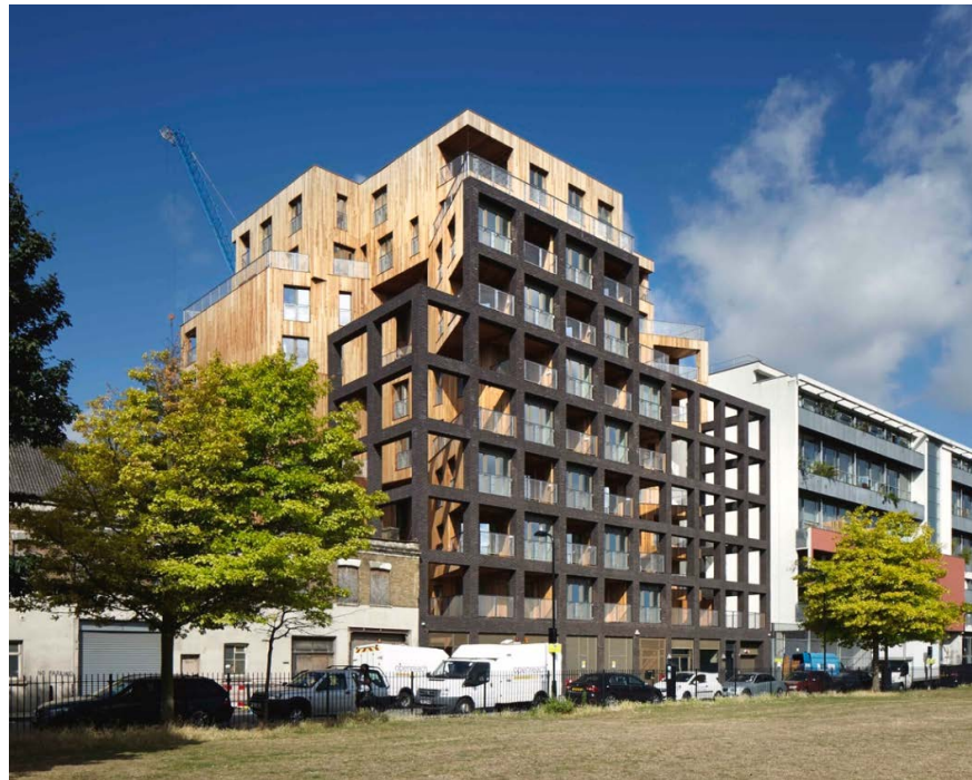
Figura 3. Jack Hobhouse. Fonte: https://www.archdaily.com.br/784367/the-cube-hawkins-brown/
